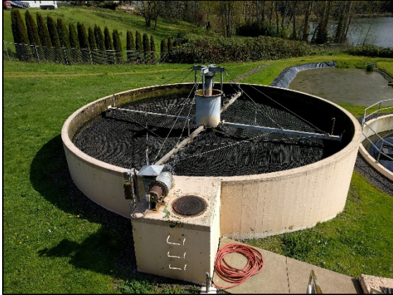
Trickling Filter at the Sewer Plant
