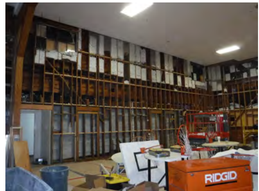
Seismic work being done in the Lundy gym.
