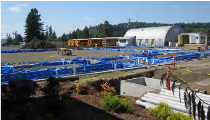
New high school gymnasium/wrestling room walls are starting to go up!
